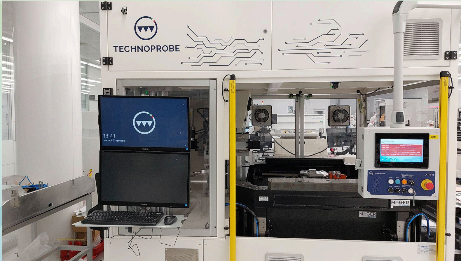
FTPA installed in TPI clean room
